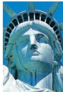
Copper reacts with oxygen in air.
