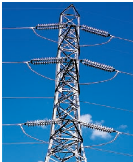
These high-voltage transmission lines are made of aluminum supported with steel cables.
